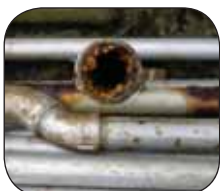
Corroded steel pipe
