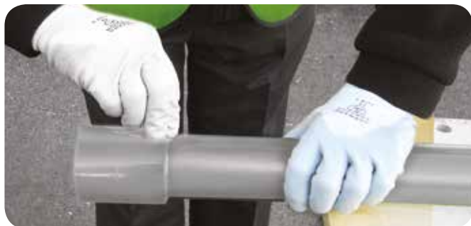
8. Using the mark previously made, check that the pipe has been fully inserted.
