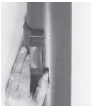
1. Position lower half of saddle around pipe.
